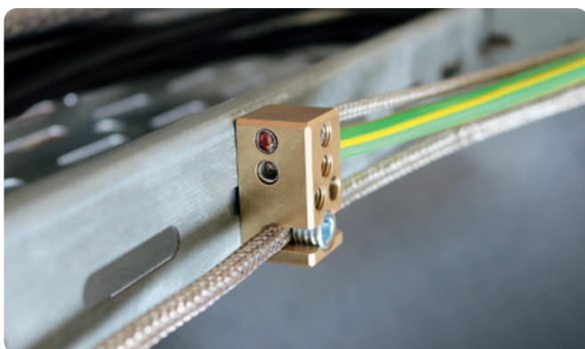
Fig. 13: Example for fastening of EmClots®
